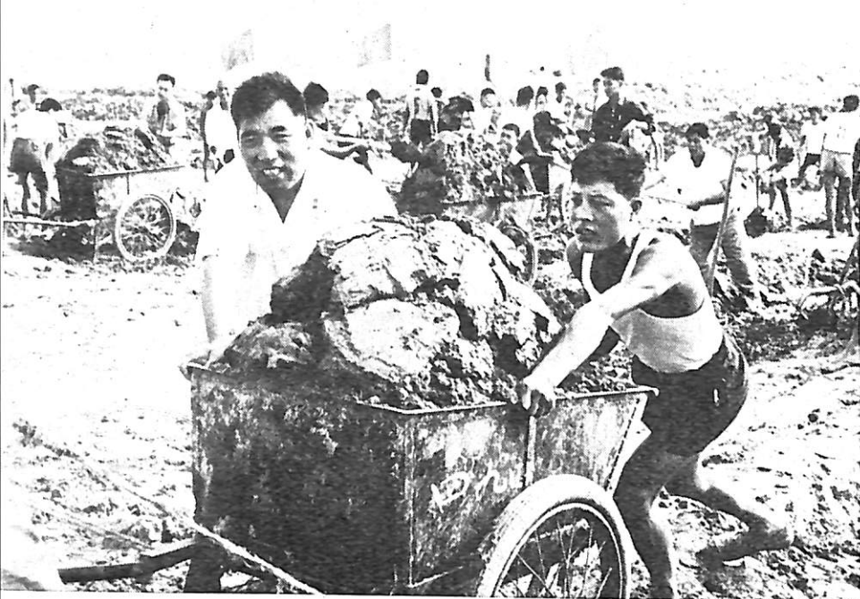
The county Party secretary working on a water conservation project.
